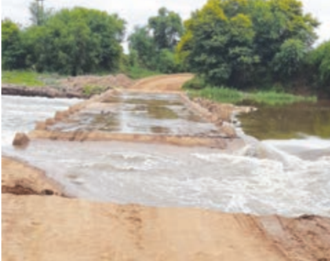
Part of the bridge collapsed and was swept away by the river's flash flood.
