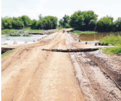
The bridge started to show cracks.
